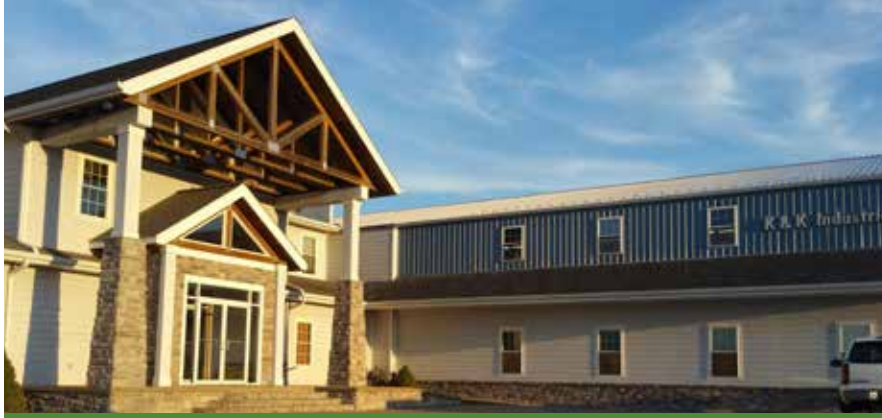
K&K Industries designs and builds custom roof & floor trusses, and pre-fab wall panels for commercial and residential use. ~ Montgomery
